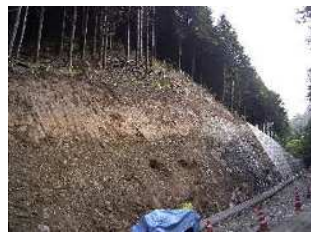
①法面清掃
