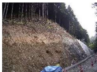
①法面清掃
